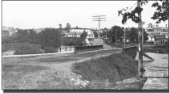
Newly built bridge over the Moose Horn River.
