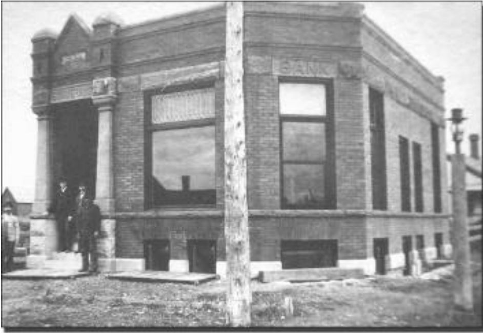
State Bank of Barnum, newly constructed in 1903
