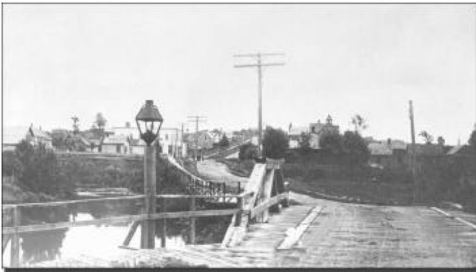
Bridge over Moose Horn River, how it looked until 1910. Viewed looking East of town.
