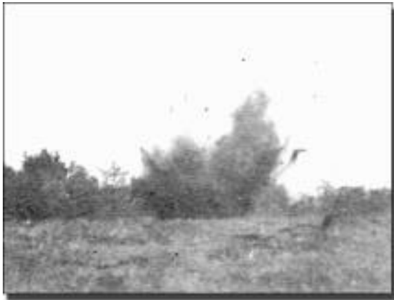
Dynamiting the stumps to clear pasture land.
